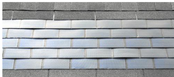
Fig. 1: Thin-film solar PV shingles. Image courtesy of NREL, PIX 13572.
